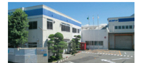
3 Kabe Plant 2-25-31 Kabe-minami, Asakita-ku, Hiroshima-shi 731-0223
